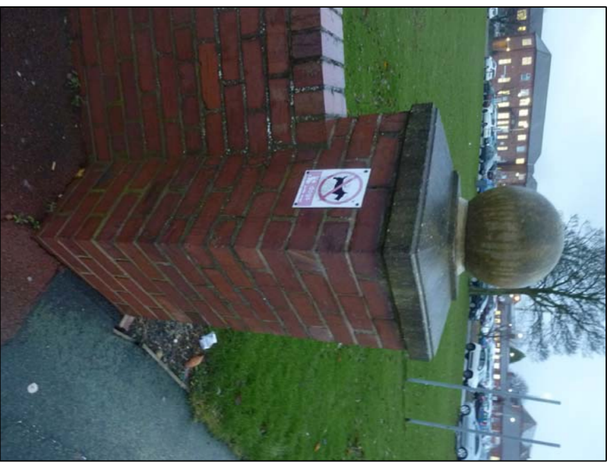
EXISTING SITE PHOTOGRAPH Existing masonry column to the east side of the site entrance off Heron Lane, column to be removed as part of demolition works, pier cap to be retained and re used to form new pier at the end of the new fence line to the east of the new Care Hub site entrance off Mackenzie Avenue
